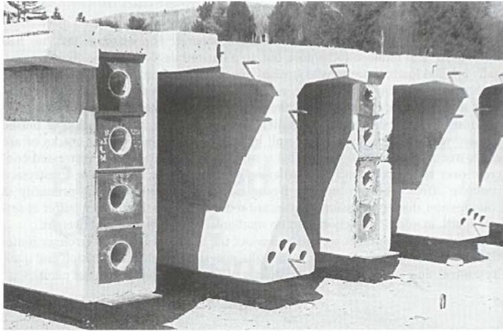
**Figure 2.** Precast bridge girder components for post-tensioning
