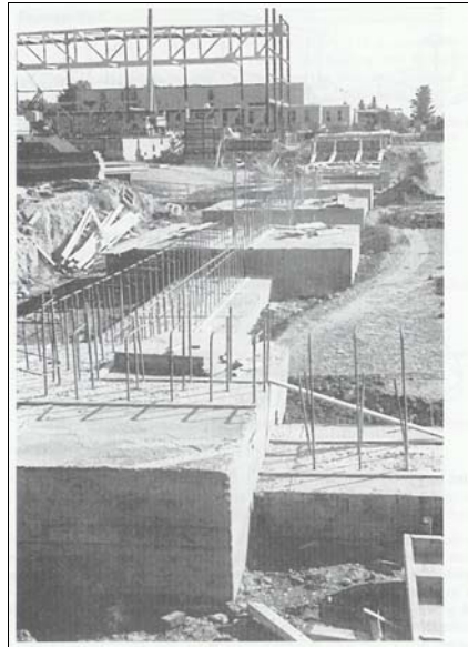
Figure 1. Column and Wall Footings
