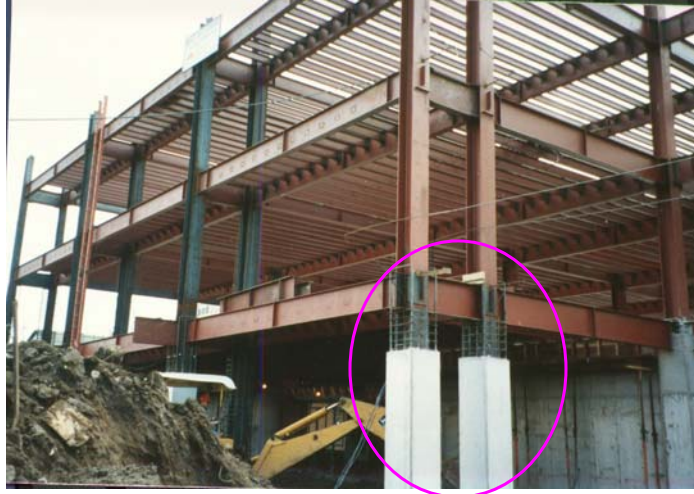
Reinforced Concrete Columns
